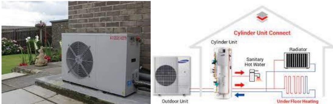
A Heat Pump works like a refrigerator in reverse – instead of cooling the inside of your fridge and emitting that heat via the back of the fridge into the room, it effectively takes heat from outside (even in cold weather) and uses that to heat hot water tank(s) to give hot water for radiators, showers etc inside the home.
